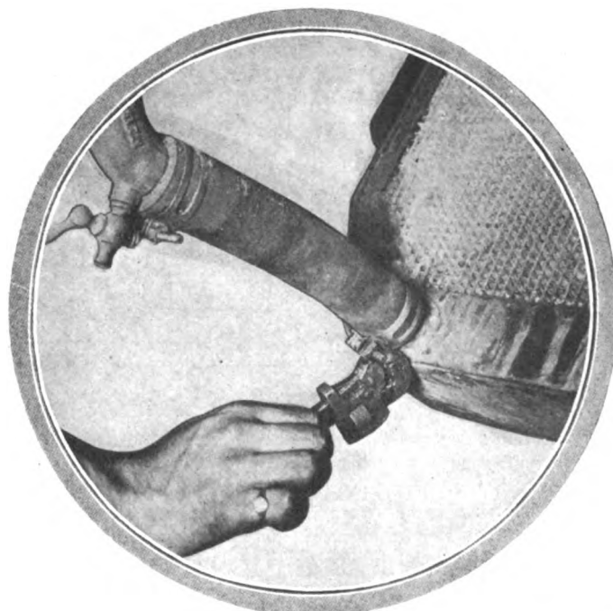
Fig. 2—Method of making a tight connection between the hose and the radiator. A metal clamp is fastened in place with a small bolt
